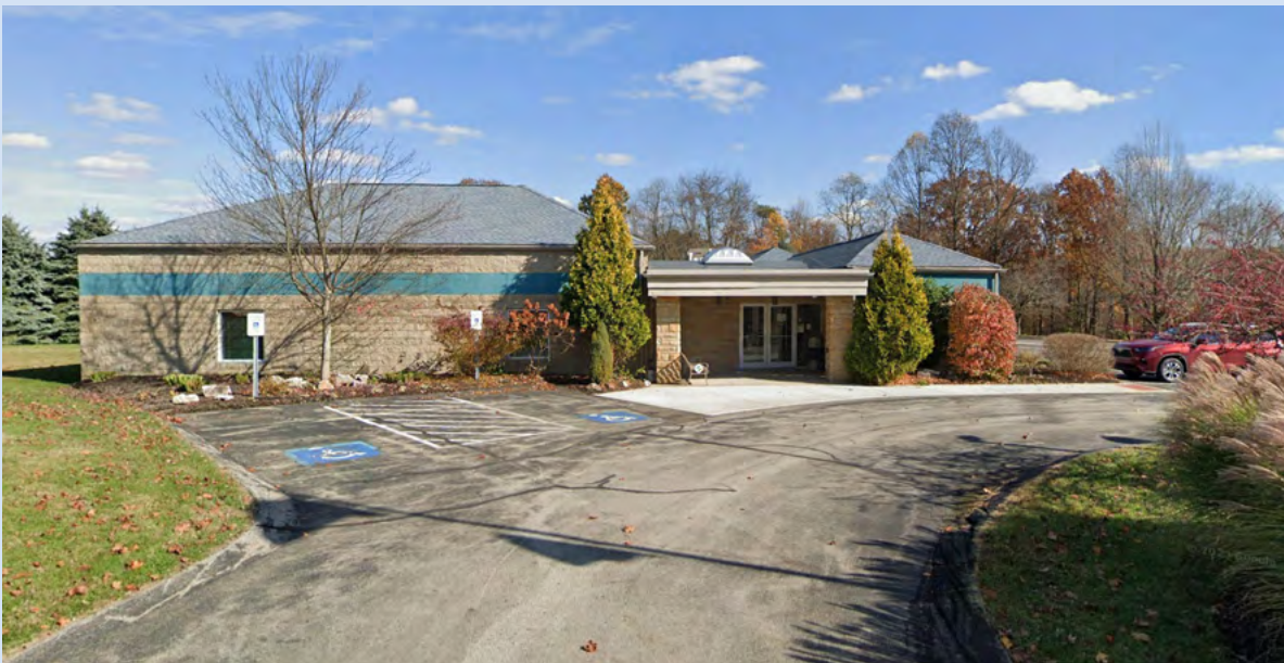
Existing Municipal Building roadway infrastructure
