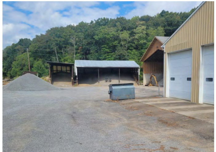
Salt storage for road management
