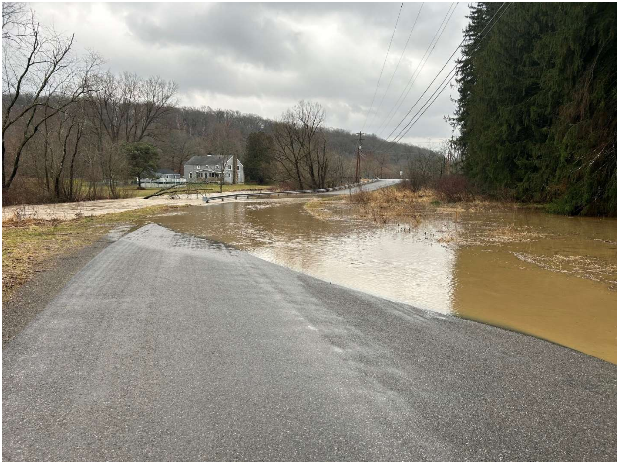
Dodds Road was flooded after heavy rains in February 2024.
